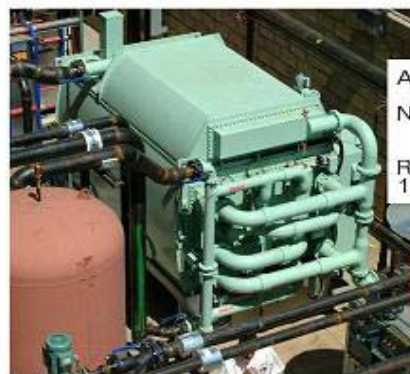
The Adsorption chiller installed in Fresno Federal Guarantee Saving Build. ( Fresno City, CA . USA )
